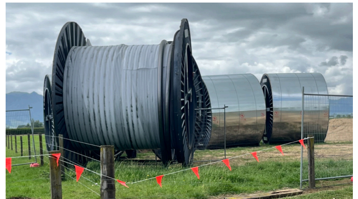
110kV underground cable drums arrive on site for installation this month.
