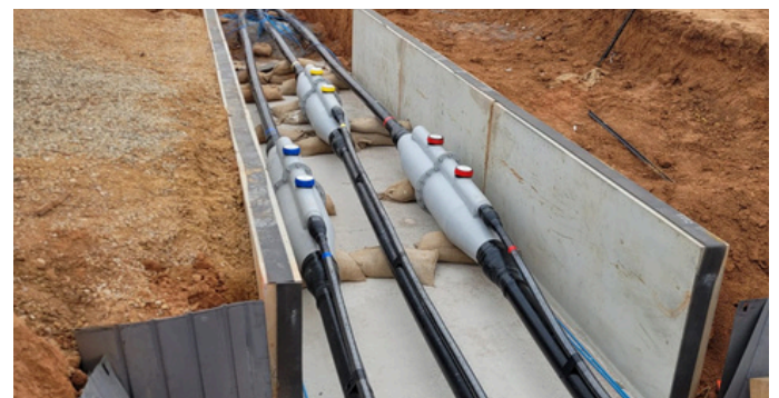
Example of an underground Cable joint Bay
